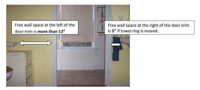
Gaining 1 ½ to 2 inches by installing swing-away hinges.
